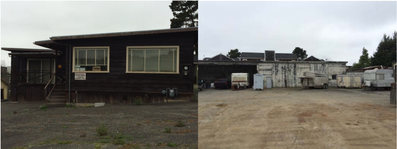
Structures to be demolished
